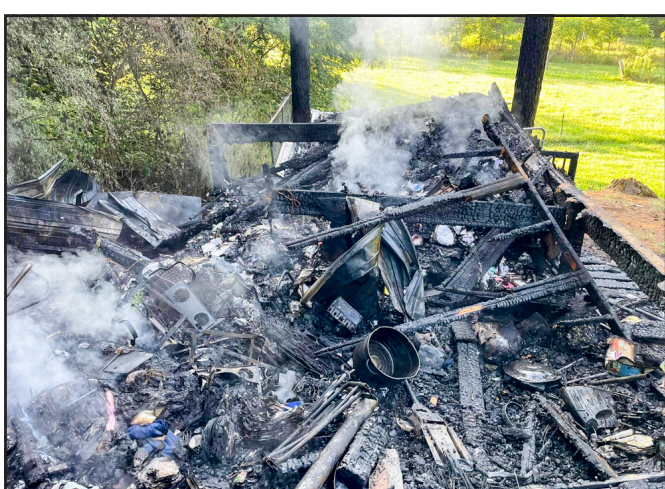
Firefighters believe this shed fire likely started from a fireworks accident in the early morning hours of July 5. Photo/Facebook
